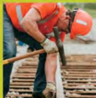
Brian Jones Track Maintenance Section Truck Driver Central Canada
